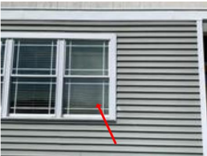
The lower right front window has a broken seal.
