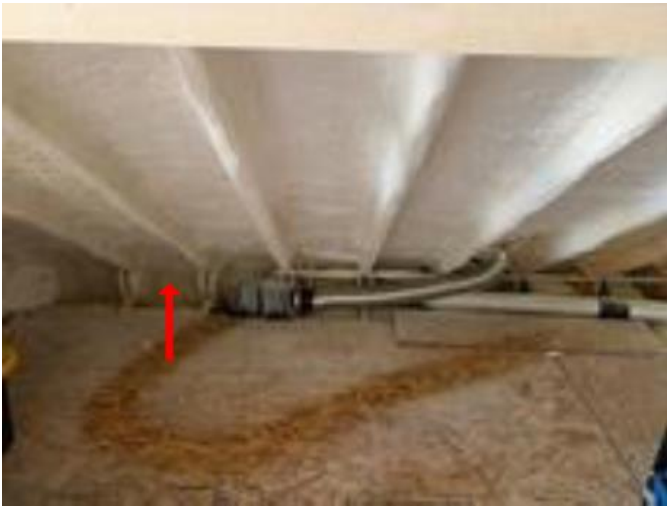
Note the soffit area ventilation is covered.
