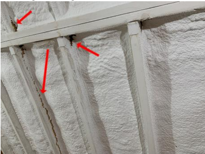
Note foam material is not attached to the structure. Exterior heat is able to penetrate into the attic space.
