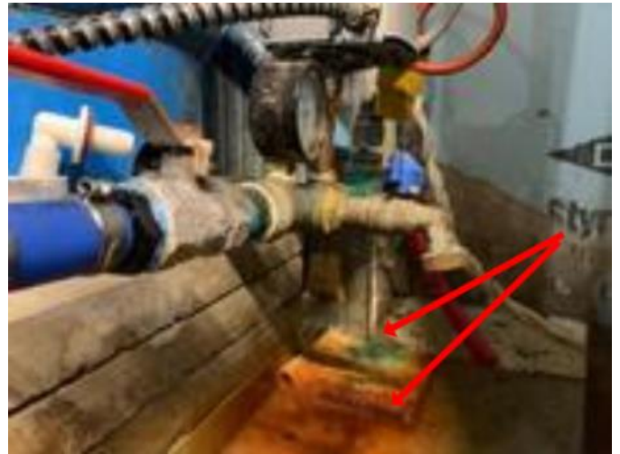
Note corrosion on floor.
