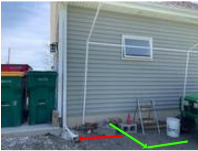
Rainwater should be directed further away from the house.
