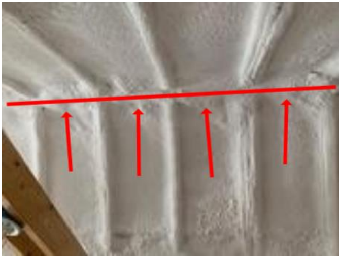
Note the ridge vent area is covered.
