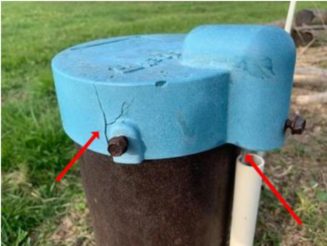
Crack noted on the well cap. Plastic conduit separated from the cap, exposing wire.
