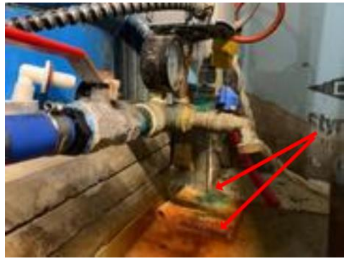
Note corrosion on floor.
