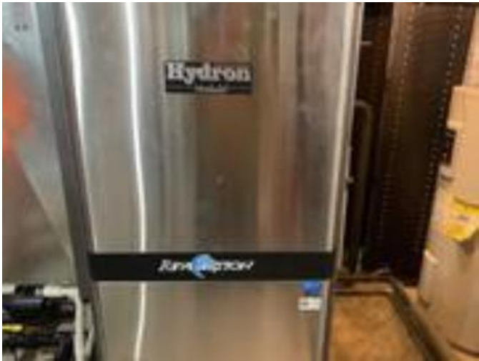
Geothermal heating/cooling system noted.
