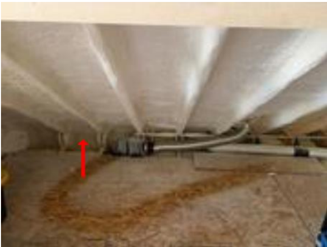
Note the soffit area ventilation is covered.
