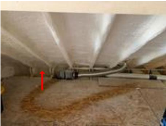
Note the soffit area ventilation is covered.
